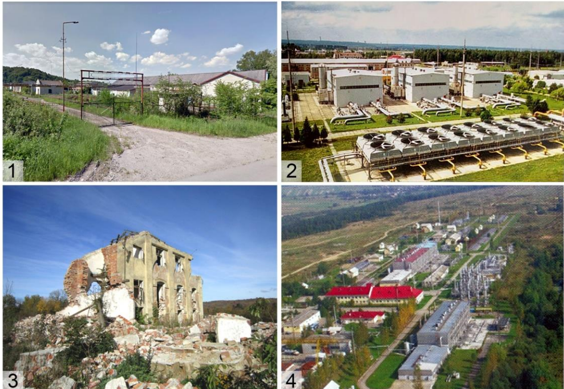
Fig. 3. 1: Oil and Gas Production Plant № 1 in the town of Boryslav, Lviv region. Source: photo by Google. 2: Bohorodchany Compressor Station in the urban-type settlement of Bohorodchany, Ivano-Frankivsk region. Source: Stepiuk & Slobodian, 2000. 3: The refinery in the urban-type settlement of Pechenizhyn, Ivano-Frankivsk region. Source: author's photo. 4: Bohorodchany Underground Gas Storage in the urban-type settlement of Bohorodchany, Ivano-Frankivsk region. Source: Serediuk & Savkiv, 2015
