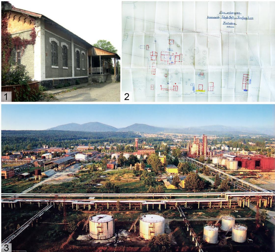
Fig. 6. Nadvirna Oil and Paraffin Factory: 6.1. Residential building. Source: author's photo. 6.2. Situational plan. Source: Stanislavsky District Mining Administration, 1934-1938. 6.3. PJSC Naftokhimik of Prykarpattia. Source: Aleksandrovych, Dutchak, Boichuk, Stelmakh, Holych & Honcharuk, 2007
